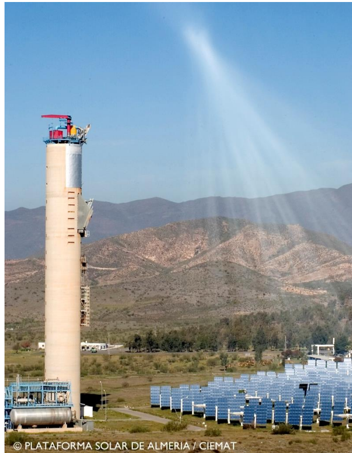
Solar tower system with the heliostats in stand-by position
