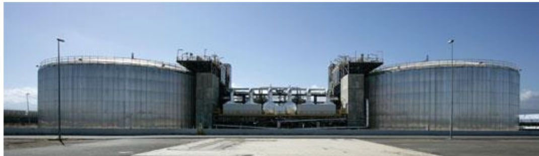
View of typical 2-tank thermal storage system with molten salts
